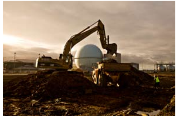
Groundworks at Dounreay (photo Dounreay Site Restoration Ltd and NDA)
